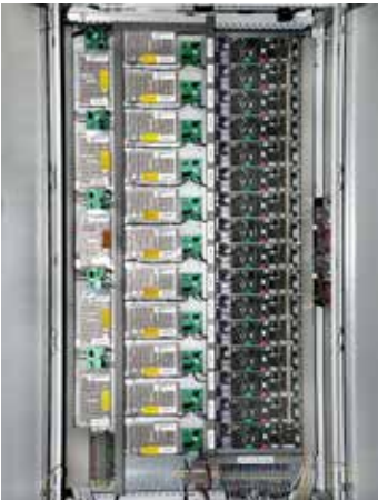
Control cabinet with power packs and zone masters that coordinate transports within the respective zone.
